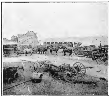
Stable Yard and Warehouse, 26th and Poplar Sts.
